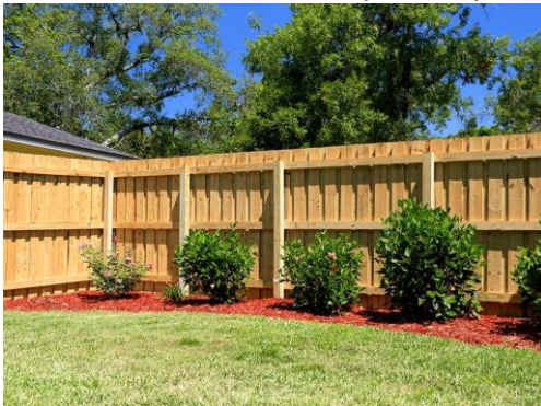
Board on Board fence
